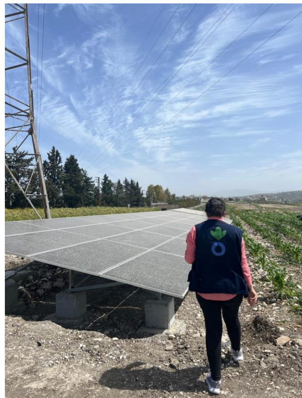
Solarization of Insariyeh pumping station
