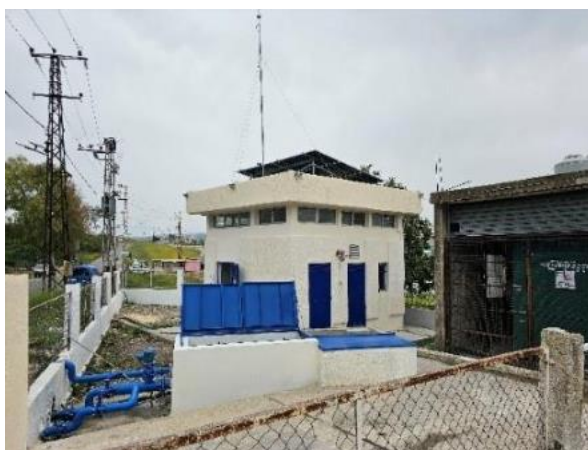
Insariyé-Adloun pumping station
