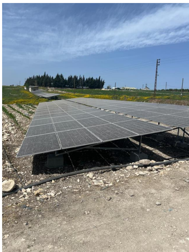
Solarization of Insariyeh pumping station
