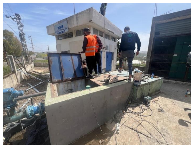
Solarization of Insariyeh pumping station
